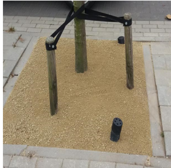
Slimme halfverharding met Jogefix i.c.m. CitySlim coating
